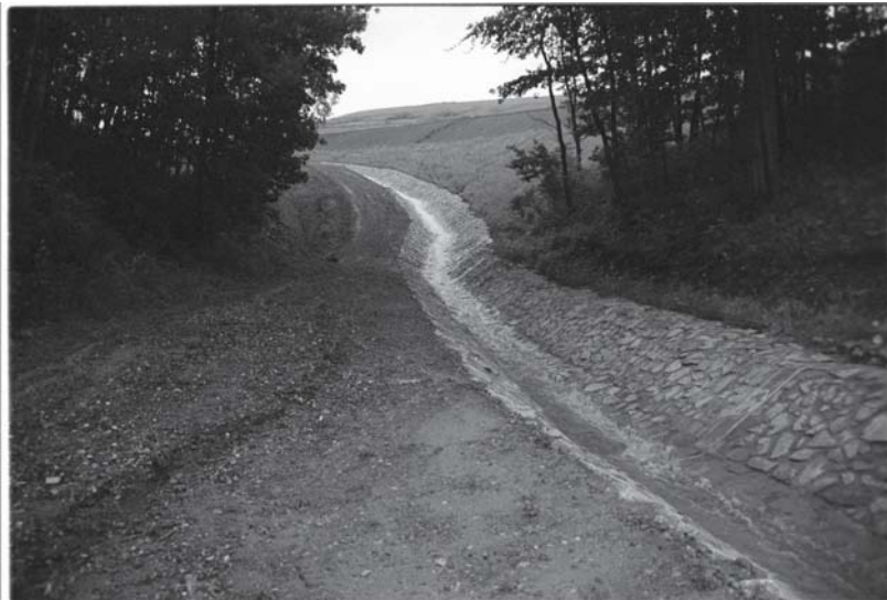
Fig. 2. Surface water runoff facility at waste rock pile 366 in Schlema.
