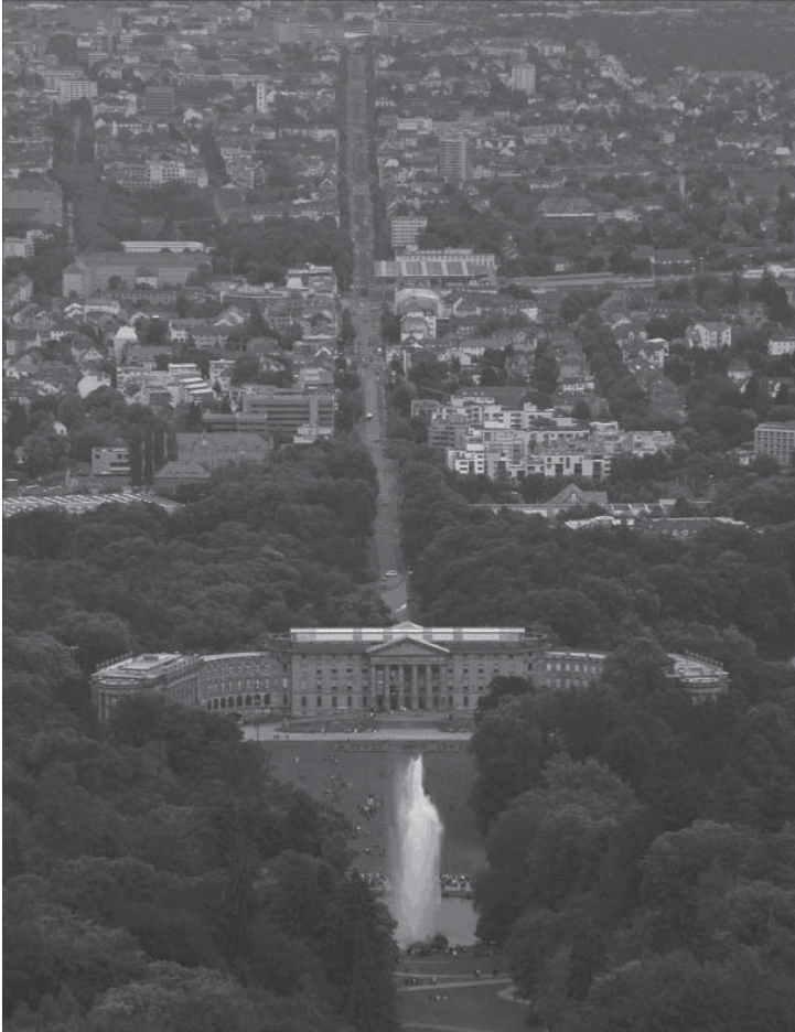
View from the Karlsberg across Schloß Wilhelmshöhe and Wilhelmshöher Allee toward the city center
