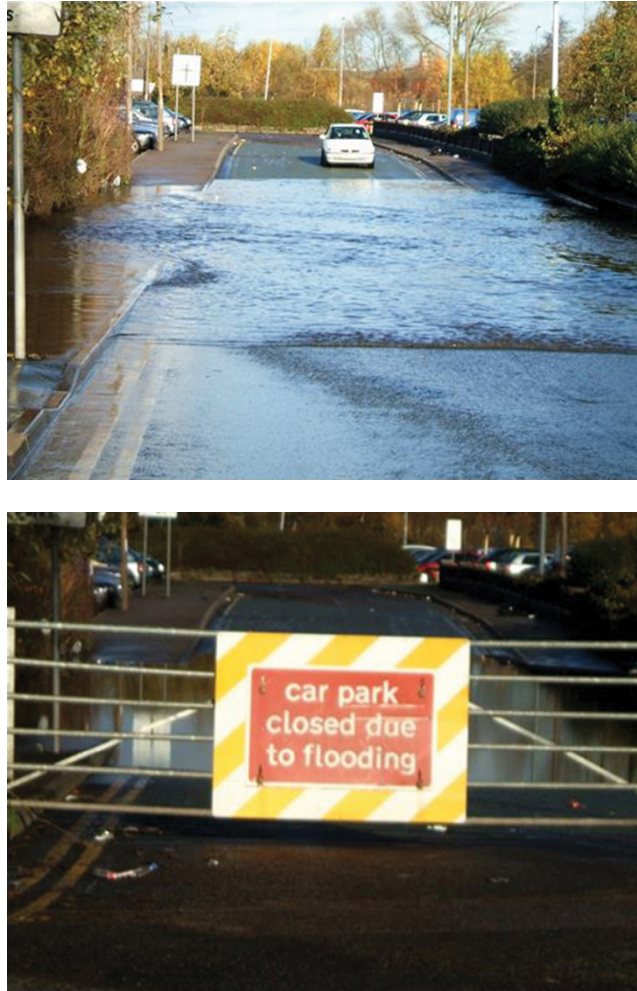
Figure 1.1 An example of a flooded car park where the impermeable asphalt surface is retaining stormwater runoff.
