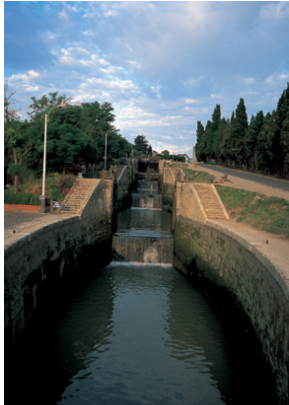
Ecluses de Fonserannes, Béziers - a flight of nine locks on the Canal du Midi
