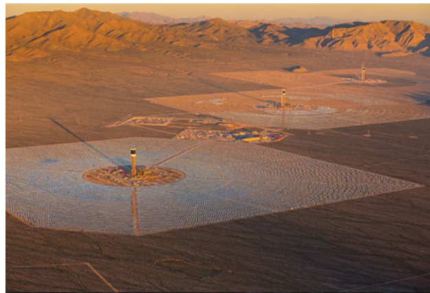
FIGURE I.13 Solar/thermal/electric generating systems in the Mojave Desert, California. Left: SEGS unit at Kramer Junction, California (2005); Right: Ivanpah installation (2013). Both systems use concentrating mirrors to produce super-heated steam to turn turbines.
