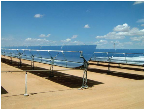
FIGURE I.13 Solar/thermal/electric generating systems in the Mojave Desert, California. Left: SEGS unit at Kramer Junction, California (2005); Right: Ivanpah installation (2013). Both systems use concentrating mirrors to produce super-heated steam to turn turbines.
