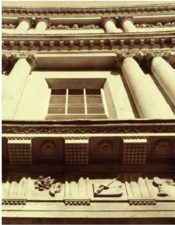
Figure 2.3 After repairs to 14 Circus during 1973/74.
