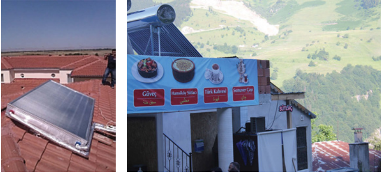
Picture 1.4 Direct solar heaters of Turkey (top figure without a tank; bottom figure with a tank).
