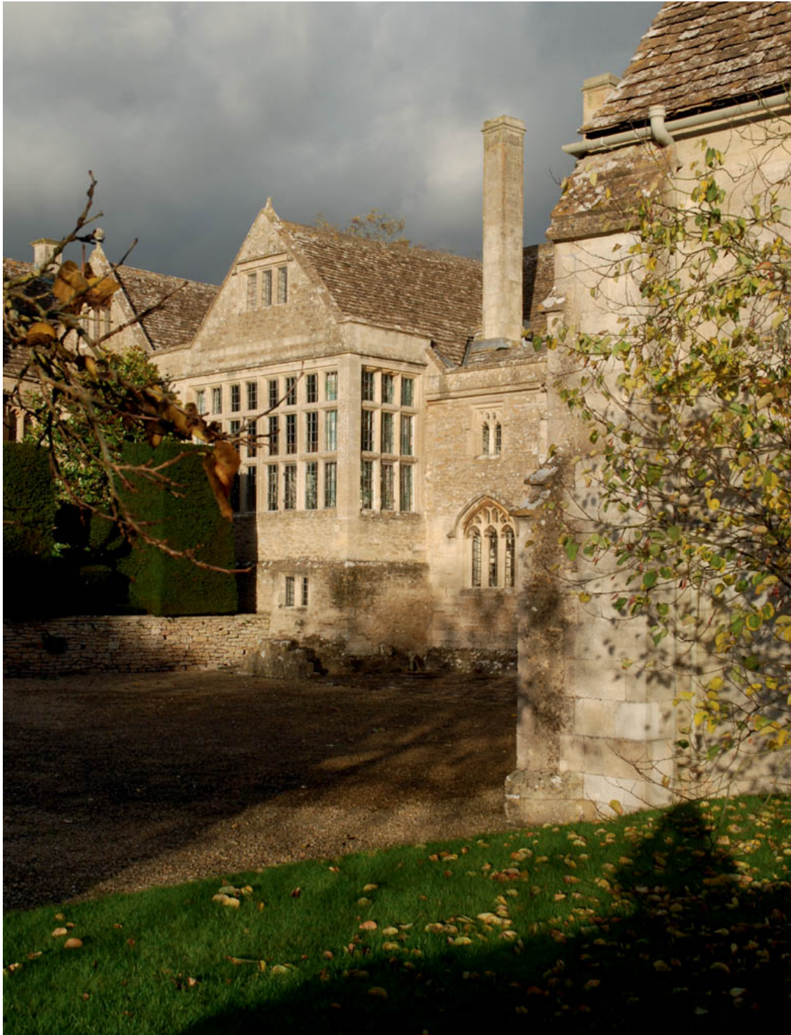
The view across the entrance court towards the huge mullioned and transomed window, added to the Great Chamber in about 1600.
