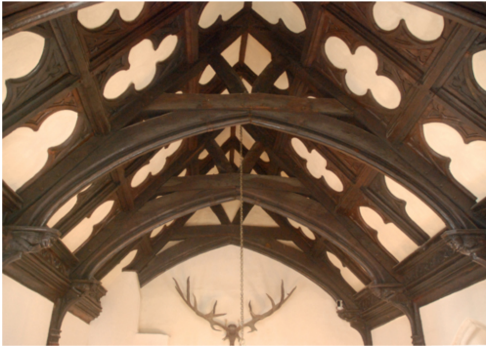
The early fifteenth-century Great Hall roof at South Wraxall, Wiltshire, a marvellous Medieval construction with a hidden meaning.
