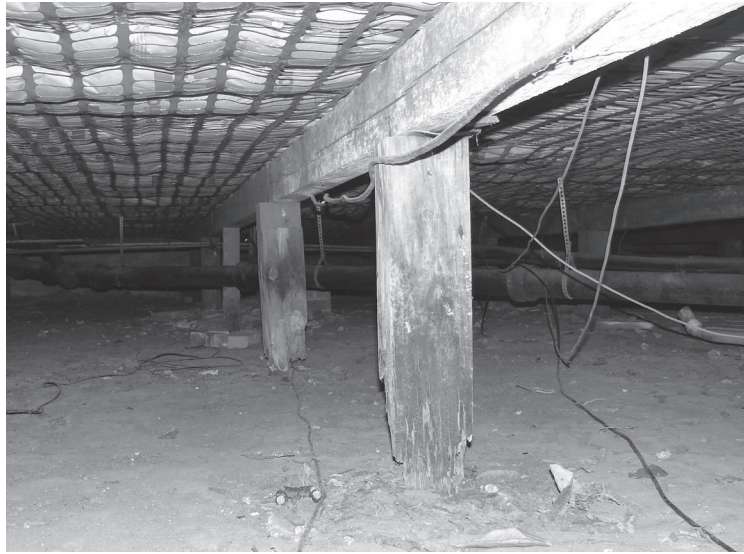
FIGURE 1.4 Deteriorated wood piers
