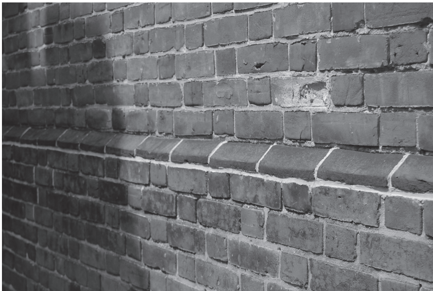
FIGURE 1.7 Brick water table
