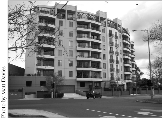
Figure 1.1: medium-rise apartment block
