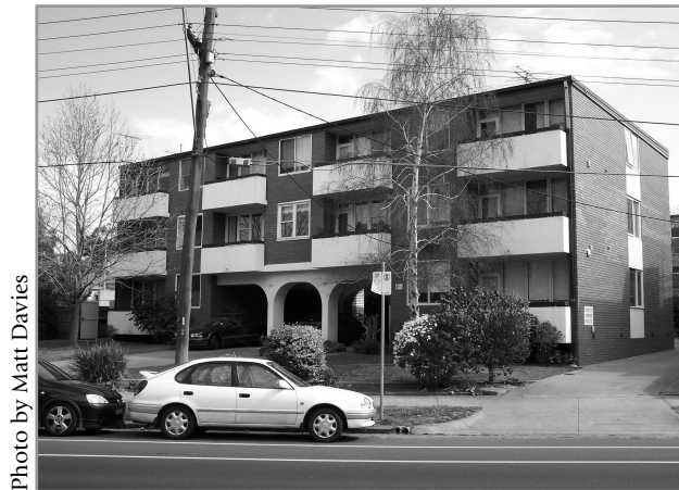
Figure 1.2: a typical low-rise apartment block
