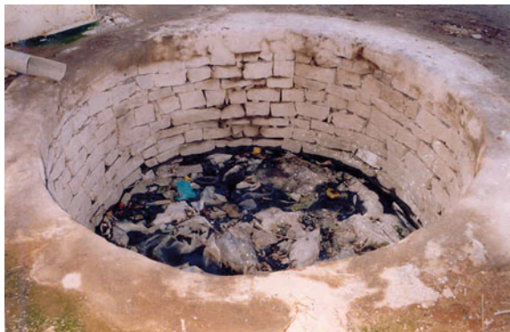
Fig. 1.2 Water contamination of groundwater due to indiscriminate throwing of solid waste into a well
