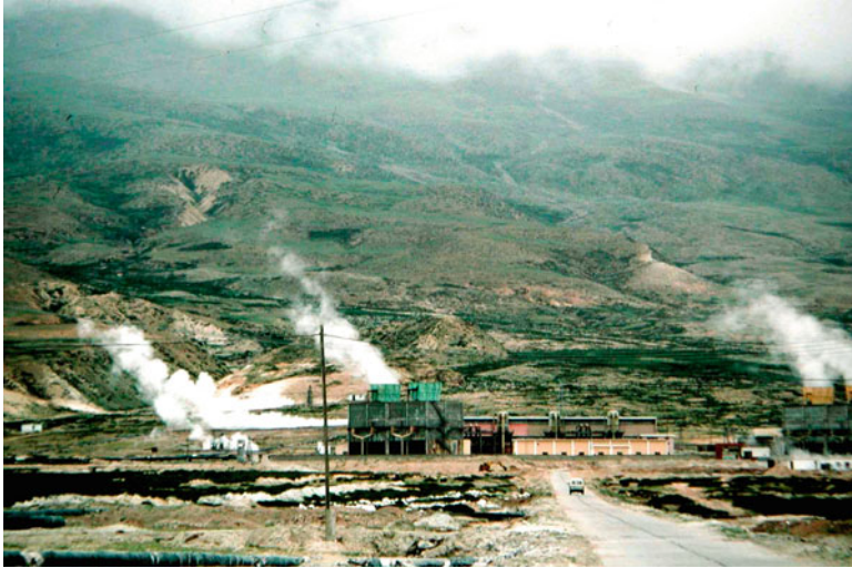
Fig. 1.9 Fault-lines and other zones of structural weakness offer preferred conduits for geothermal heat flow that leads to talik formation in permafrost. At Yangbajing on Tibetan Plateau, geothermal heat has been tapped for decades as an energy source for power generation
