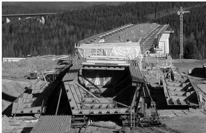
Fig. 1.1: Assembly of Haseltal road bridge near Suhl, Germany
