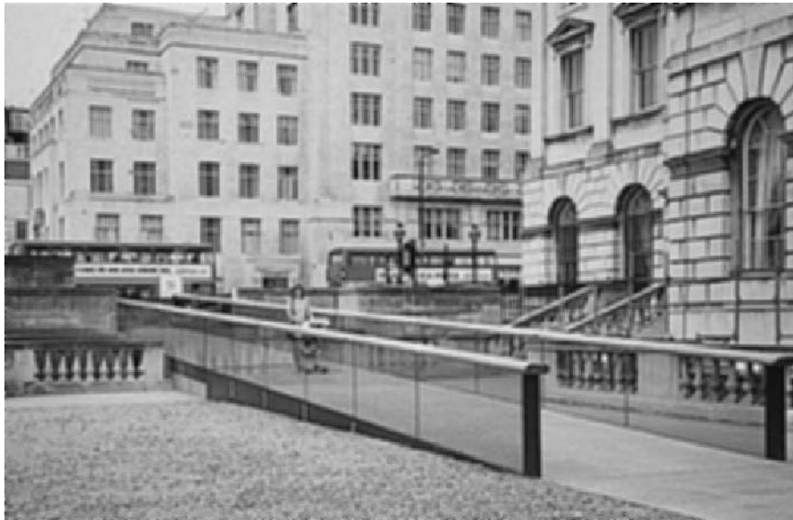
Figure 1.2 Access to historic buildings can be improved with sensitive, well-designed alterations.
