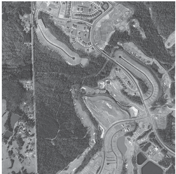
Sun City Peachtree, a 1,726-acre senior community, currently under construction 35 miles south of Atlanta, Georgia.
