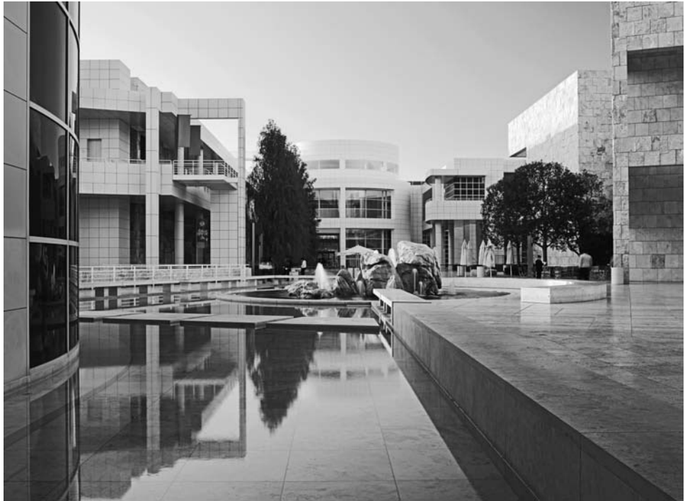
FIGURE 1-8 This is one of many gardens at the J. Paul Getty Center. All of them are over various structures used as garages, shipping and receiving facilities, storage areas, mechanical rooms, and portions of the scholars' libraries and studies.
