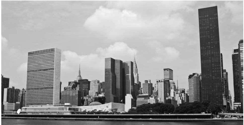
FIGURE 1-1 Gardens at the United Nations, viewed from the East River, illustrate extensive portions built over the FDR Drive.
