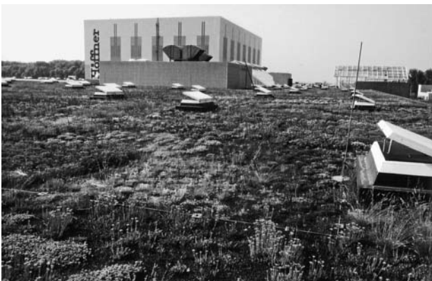
FIGURE 1-11a Utilization of roofs for stormwater management systems at a manufacturing plant. (Photo: re-natur, 24601 Ruhwinkel, Germany)
