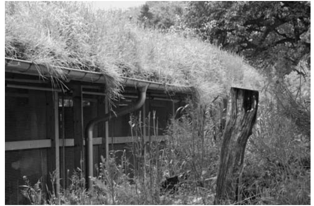
FIGURE 1-12b A traditional vegetated roof insulates the coop at a Swiss poultry farm while also helping to integrate the roof into the surrounding rural landscape.
