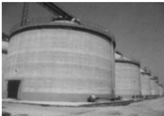
Fig. 1.2 Reinforced concrete grain silo used for the storage of paddy in China.
