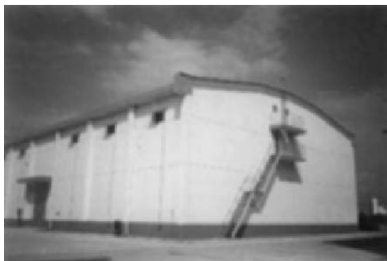
Fig. 1.1 Soviet-style warehouse for the storage of paddy and milled rice in China.
