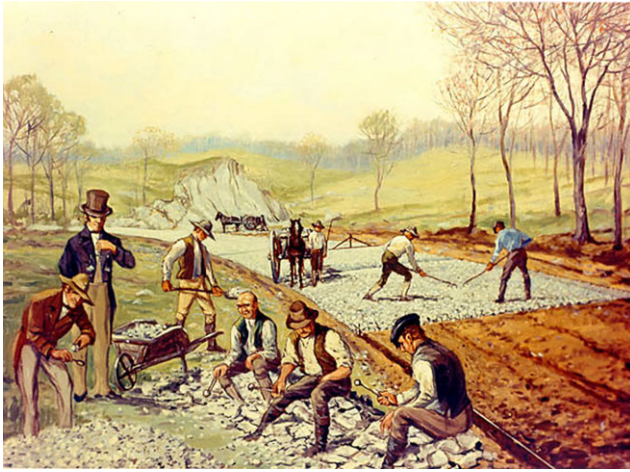
Abb. 1.6 Bau einer Makadamstraße: Rakeman, Carl: Construction of a macadam road at the time of John Loudon McAdam, 1823, Federal government of the United States
