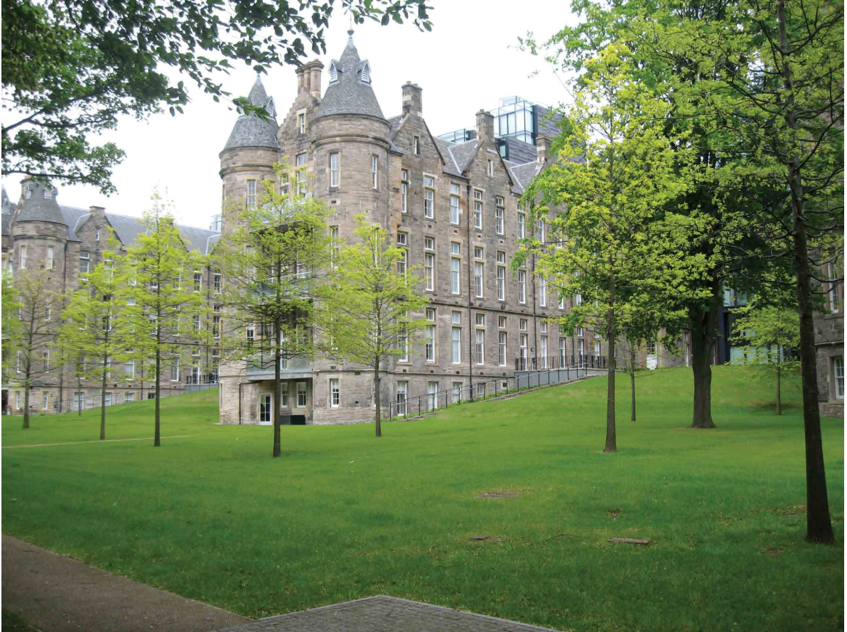
2.4 Nineteenth-century pavilion-style hospital, Edinburgh Royal Infirmary (now converted to apartments), Edinburgh, Scotland.
