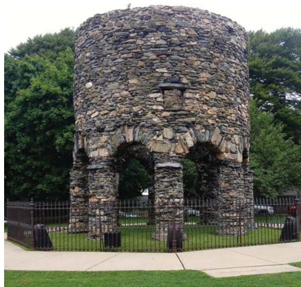
Figure 4 The Newport tower has been radiodated from its mortar to the late seventeenth century, confirming a Colonial-era construction (By owner's permission)
