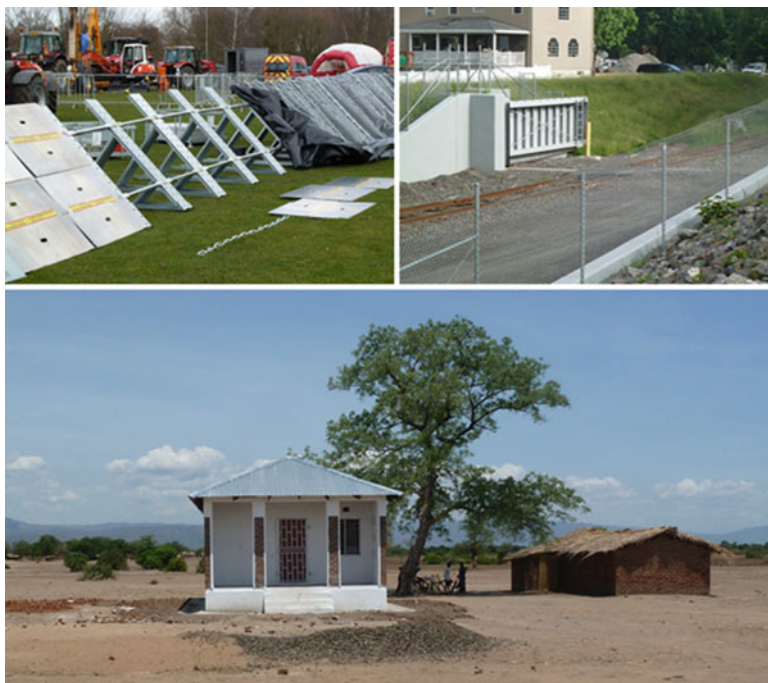
Fig. 1.3 Clockwise from top left: temporary barriers on display at an exhibition of flood emergency response equipment (UK), flood closure gate in a levee system (USA), flood resilient temporary grain store as part of a community-based flood warning system (Malawi)
