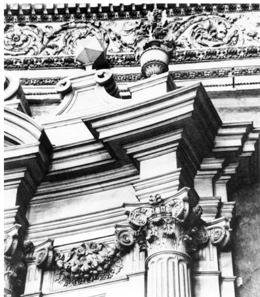
Figure 1.9. The icosahedron and other polyhedra often appear as decorative elements in Baroque architecture; here, the church of Santissimi Apostoli by Borromini.
