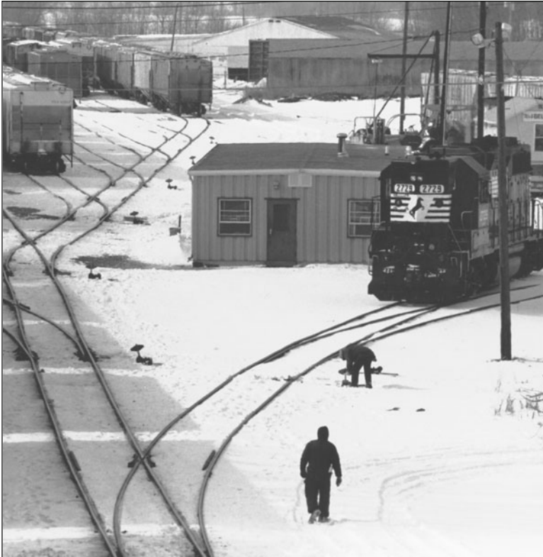
Fig. 1.6. Snowfall in rail yards brings a multitude of problems including frozen switches, frozen couplers, and discomfort and danger to work crews. Here, two heavily clad yard workers are trying dig out the frozen, snow-clogged switches so the yard's switcher can move out and go to work.
