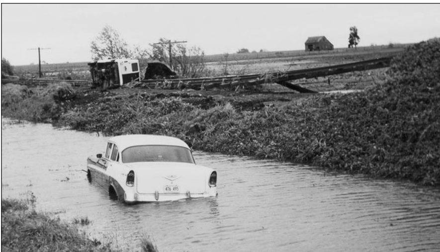
Fig. 1.3. Sometimes locally heavy rains produce 6 to 10 inches of rain in a few hours, resulting in flash flooding that causes sudden washouts of roadbeds and bridges, as seen in this Missouri branch line. A May rainstorm produced 11 inches of rain in 6 hours, resulting in these massive damages, with vehicles swept off a highway that paralleled the line.
