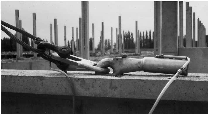
Fig. 2.6 Round-headed transport anchor
