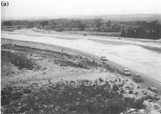
(a) Fig. 6.10. Advancing undular surge in a Durance River (France) power canal (courtesy Electricité de France)
