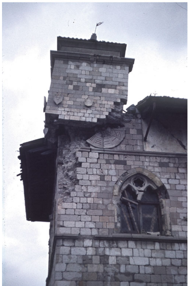
cal times. (b) Sideward displacement of the mayor's house in the medieval township of Venzone (northeast Italy) during an earthquake 50 years ago. The small roof tower stayed almost at its old place.
