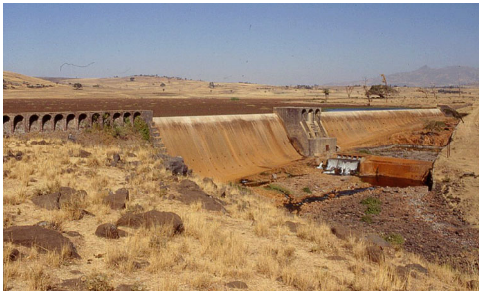
Fig. 1.6 The Aba Samule Reservoir on the Akaki River, south of Addis Ababa ( 8^{\circ}47'15''\text{N} – 38^{\circ}42'18''\text{E} ). The dam was constructed in 1939 but a few decades later it was completely filled with sediment
