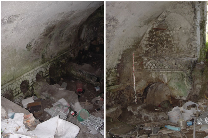
Pozzuoli, Masseria Caleo farmhouse. Remains of the Roman ninfeo reused inside the cellaio and remains of walls in opus reticulatum reused in the structure of the furnace (picture by R. Picone)
