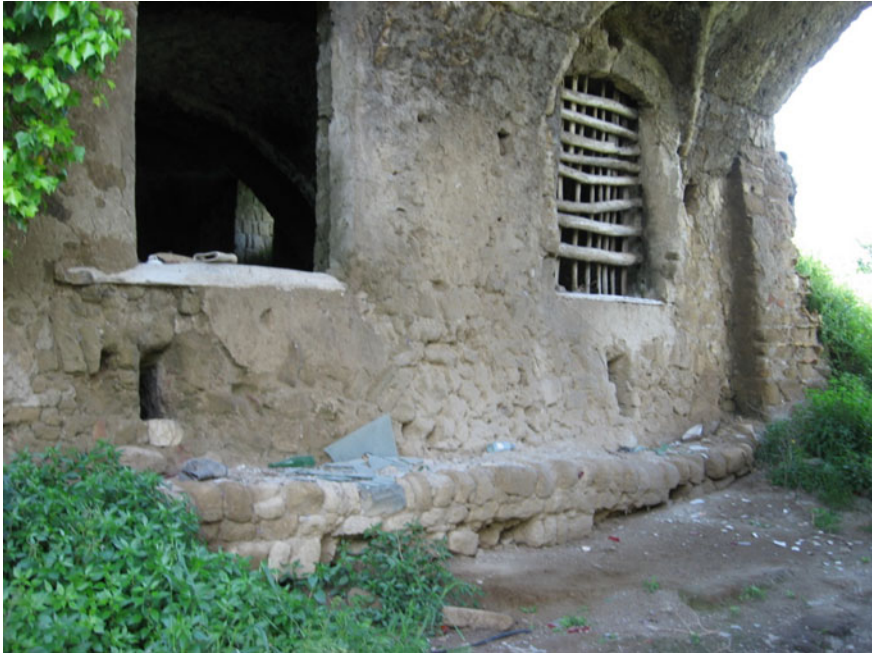
Pozzuoli (NA), Frà Vecchia farmhouse (XVIII sec.). Exterior view of the “order to sit”, where the harvest was positioned (note the presence of the wooden elements used instead of the iron for the closing of the compartments-window)
