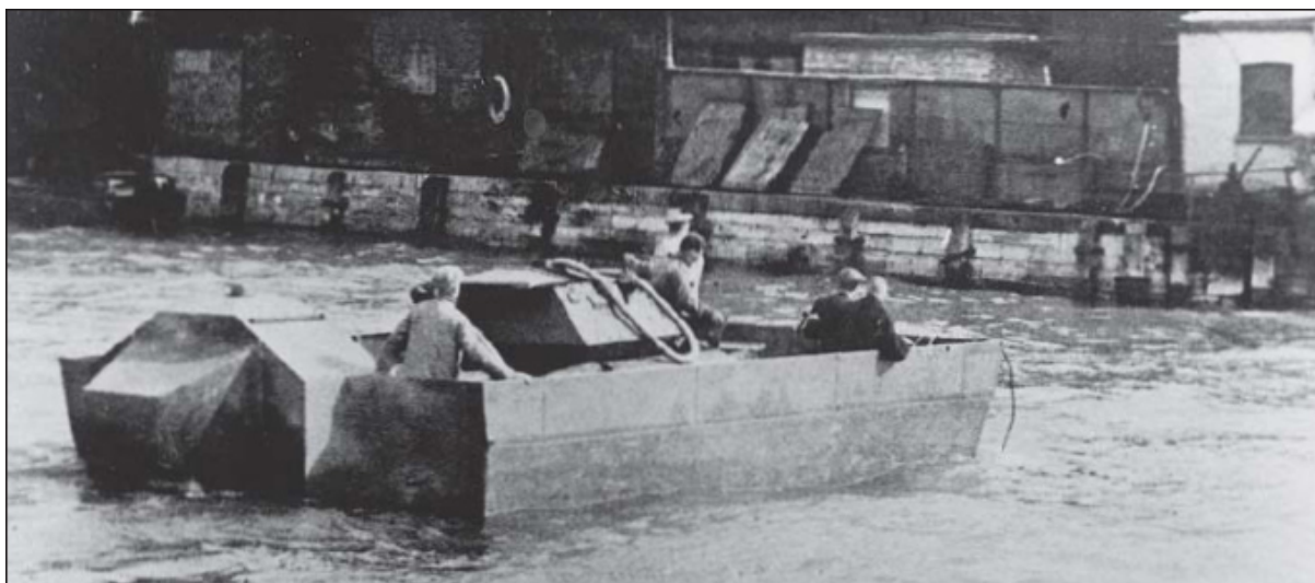
With the turret of a Covenant tank just visible above the bulwarks, a prototype of the 17-ton Lighter makes its way carefully from ship to shore in Portsmouth Harbour. The helmsman is in the housing at the back with the outboard drive in an extension at the rear.
