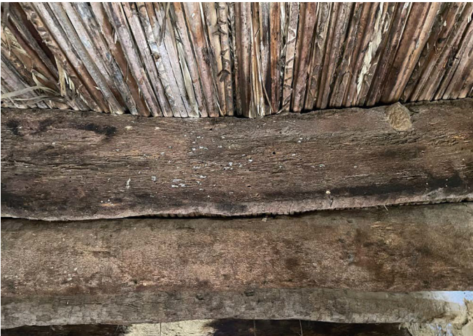
Fig. 23.10 Particular saprophyte insect attack, visible through big exit holes on the surface (author's photo)
