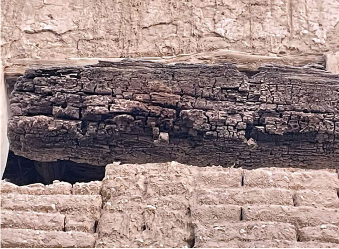
Fig. 23.9 Particular saprophyte fungi attack, well visible through cubic or brown rot (author's photo)
