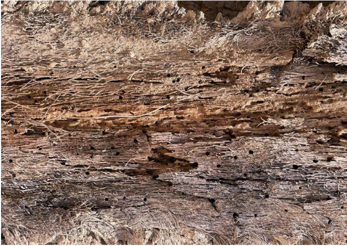
Fig. 23.11 Particular saprophyte insect attack along the core of the beam, well visible through small exit holes on the surface. Probably, the insect attack also occurs with fungi attack (author's photo)
