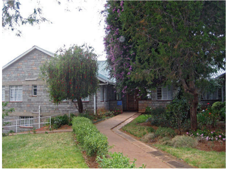
Fig. 1.1 The bright, clean, welcoming entrance to CURE's Pediatric Orthopedic Hospital in Kijabe, Kenya
