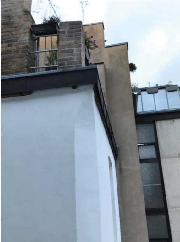
Figure 1.5 Wall from outside (private photo).
