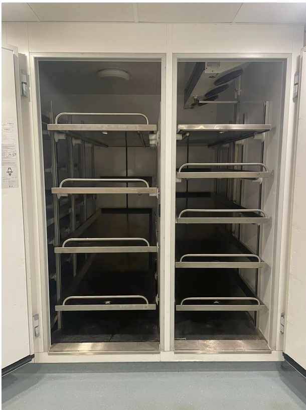
Fig. 1.13 An example of body storage is shown here, with a refrigerated compartment containing horizontal tiers of roll in/roll out trays. The tray travels with the body during the stay in the mortuary. The trays and bodies are usually arranged in tiers of three to five and vary in size to accommodate bariatric bodies. The units have doors at the head and feet ends. They are run at a temperature of 4 °C (40 °F) or freezer temperature of -20 °C (-4 °F)
