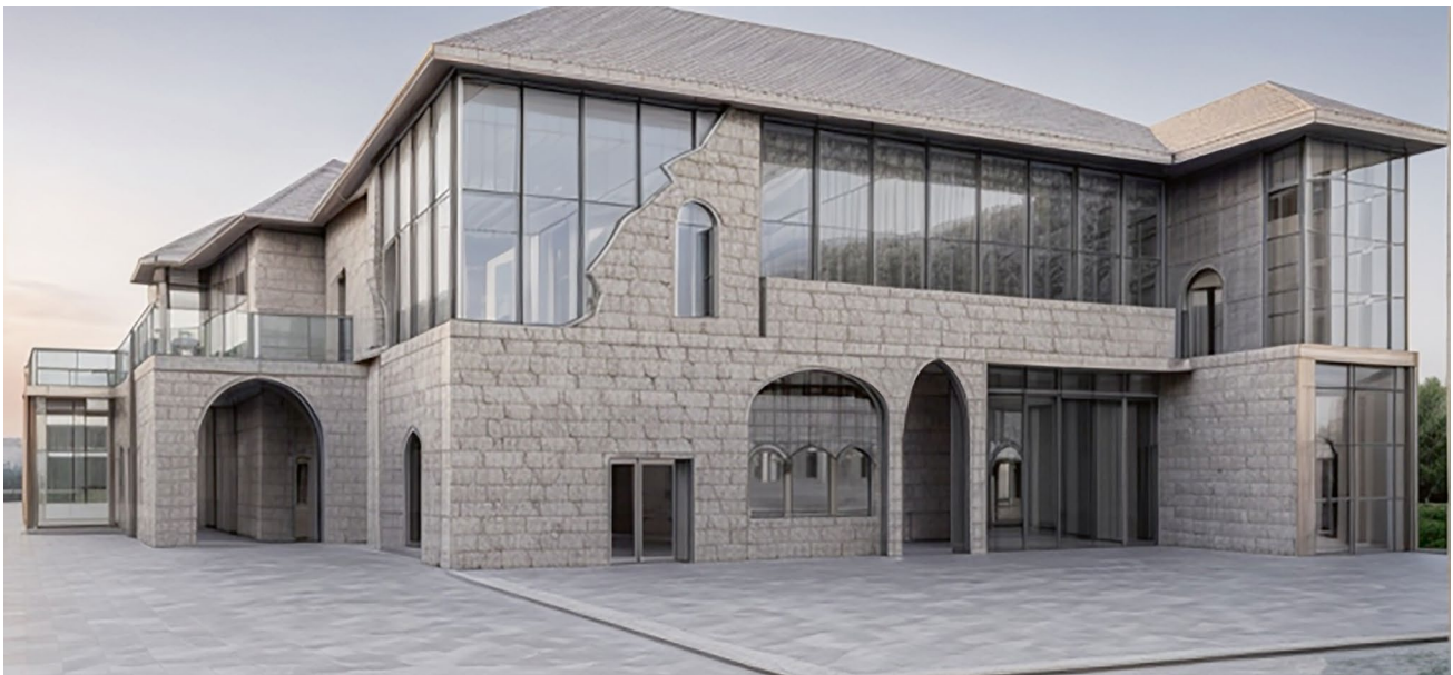
Fig. 14 Al-Nouri historical building in Tripoli, Lebanon: after developing while preserving architectural identity (Author, 2023)
