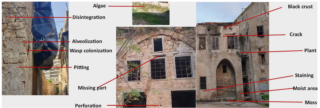
Fig. 13 Al-Nouri historical building in Tripoli, Lebanon: Condition before development (Author, 2023)
