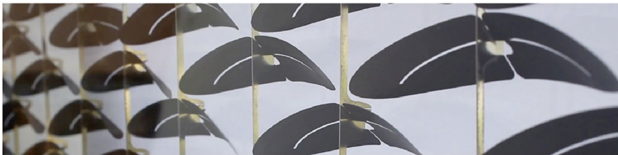
Fig. 1.3 Invert auto-shading windows [P18], self-shading project. (Source: photo by Pinkelephante (2018), CC-BY-SA-4.0, via Wikimedia Commons. Available at: https://commons.wikimedia.org/wiki/File:Invert_Shading_System.png (Accessed 12 October 2023))
