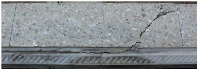
Figure 4. Longitudinal cut through the upper chord of specimen C70-1,00-300-C30/37-Ø15/18h-1.
