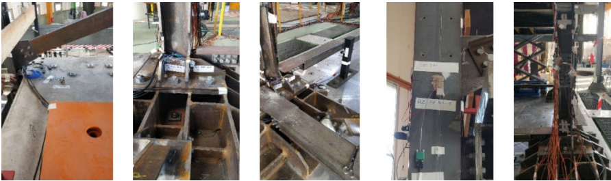
Fig. 5. The instrumentation and measurement devices installed on the mock-up.
