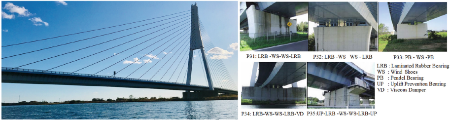
Fig. 8. Shin-Nakagawa cable-stayed bridge ( 36^{\circ}21'25.81''N , 140^{\circ}33'28.04''E ) and layout of wireless sensor network [6].
