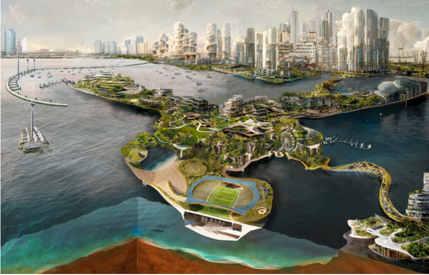
Fig. 2 Key features of S^2FS^2 , a hybrid solution combining floating structures with land reclamation featured by low-rise recreational, public and green functions on floating platforms on the foreground, and high-rise buildings on reclaimed land on the background
