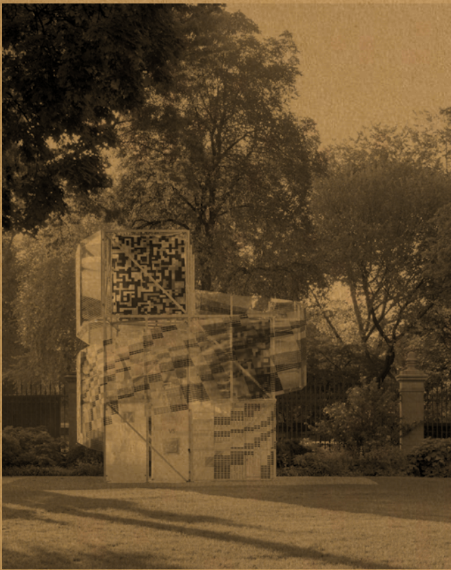
[Fig. 1] SmartWrap Pavilion, Cooper-Hewitt National Design Museum, New York City, KieranTimberlake Associates (2003). Photo by Barry Halkin.
