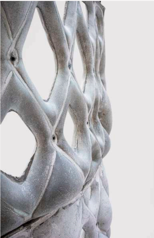
[Fig. 34] An elevation view from the other side showing how the form transition from the bottom to the top produces a stable structure. Photo by the author.
