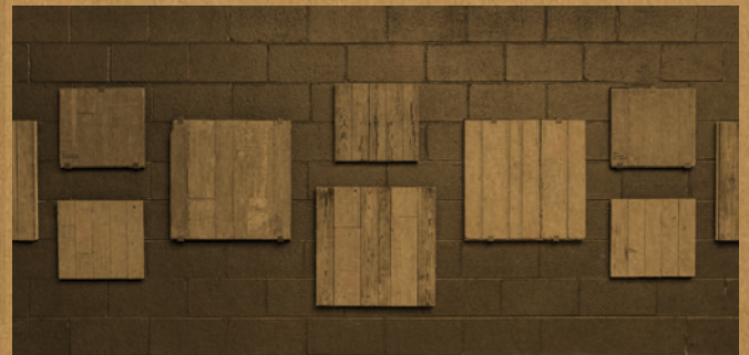
[Fig. 5] Board-formed concrete mockups of the Pendleton West complex, Wellesley College, Wellesley, Massachusetts, KieranTimberlake Associates (2017). Photo by KieranTimberlake Associates.
