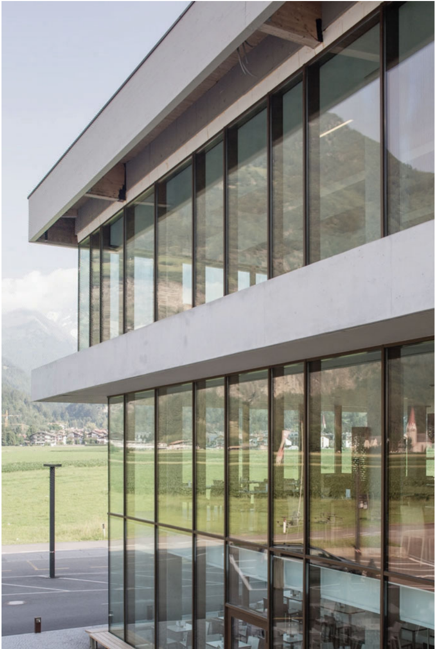
Fig. 1.1 Christoph Mayr Fingerle, Cascade Swimming Centre, Campo Tures (Bozen). Role of “transition” between internal and external spatiality of the envelope, understood as a modular apparatus warped from the load-bearing framework towards the glazed surfaces, inserted in the horizontal perspective composition. © Courtesy of Schüco
