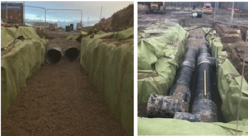
Fig. 5. Construction of perforated pipes within attenuation trenches.
