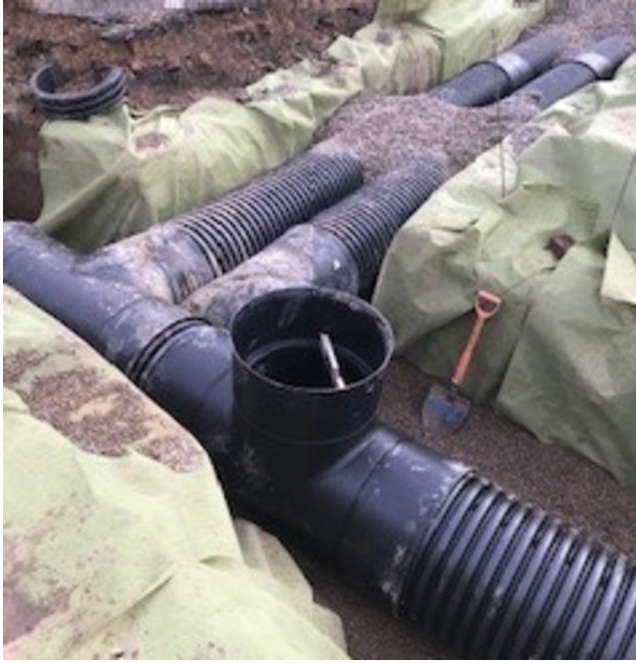
Fig. 6. Connection of attenuation pipework to maintenance chamber.
