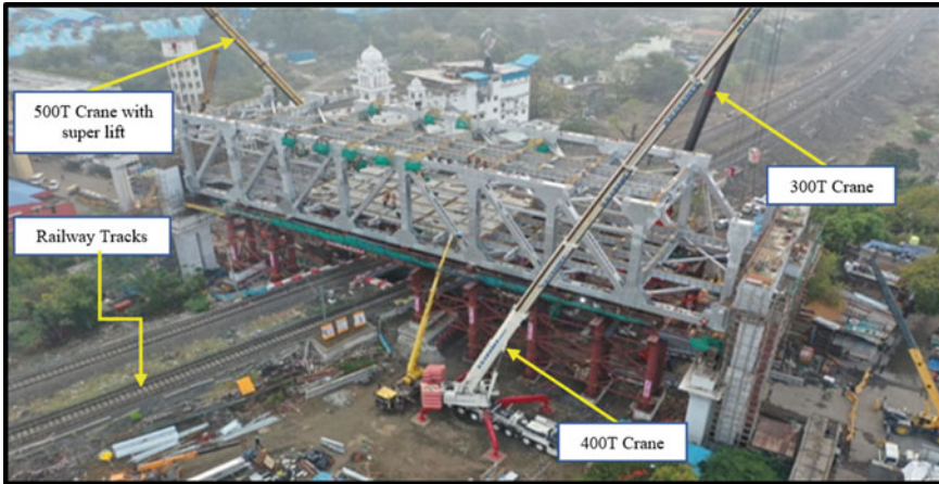
Fig. 8 Use of 3 nos. of cranes for parallel erection of members
