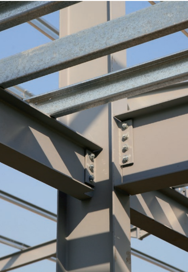
1.17 Connections for transferring shear and/or normal forces between beams and columns.
