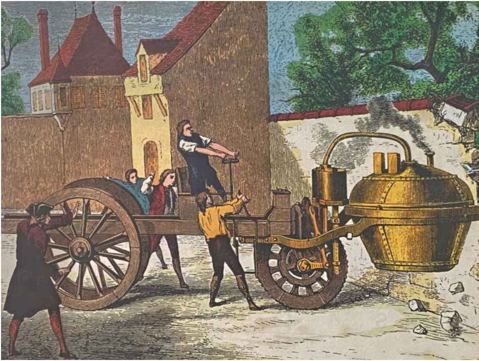
Figure 3 Cugnot's Steamer ("Fardier de Cugnot"), tested in Paris in 1770.
