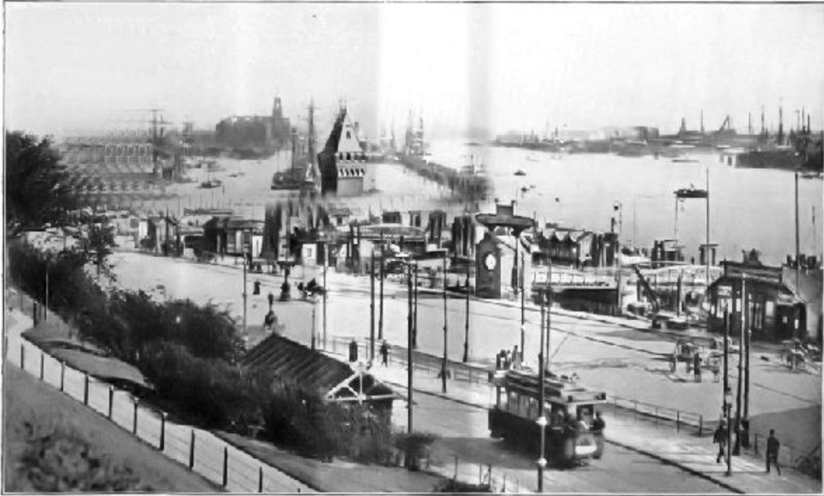
A HANSE CITY—HAMBURG, ALONG THE WATER-FRONT
