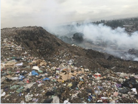
Figure 1.6 Landslide at the Koshe dumpsite in Addis Ababa. (a) Slope failure at Koshe. Source: Photo taken by author from site visit by SWIS. (b) Residential houses next to the failure site. Source: Photo taken by author from site visit by SWIS.
