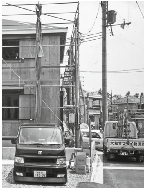
FIGURE 1.7 The North American wood light frame building system is now used extensively in Japan, where its resistance to earthquakes makes it most practical. Source: Photo by Rob Thallon
