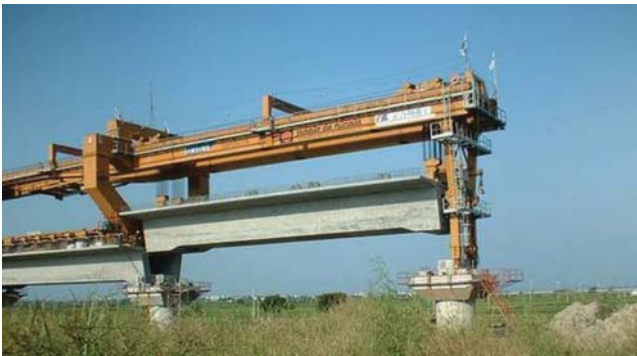
Figure 1.2 Span by span isostatic solution: China, China Railways (Courtesy of China Railways).
