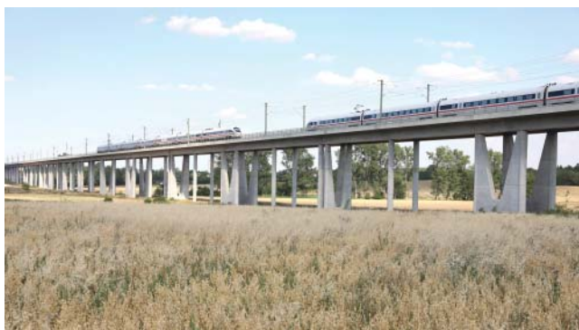
Figure 1.3 Gänslebachtal Viaduct (schlaich bergermann partner sbp), Germany, DB Netz AG (Source: Störfix).
