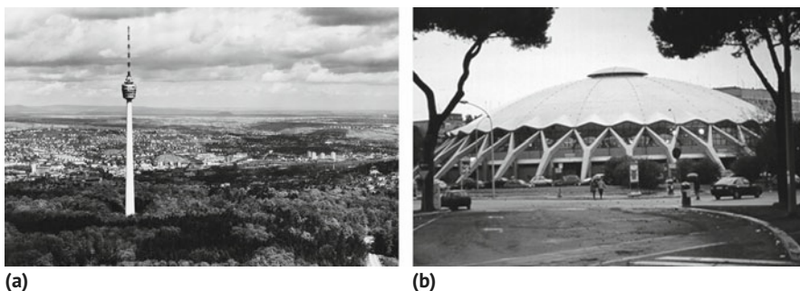
Figure 1.1 (a) Stuttgart television tower, from Kleinmanns and Weber (2009) , photography: Landesmedienzentrum Baden-Württemberg: Albrecht Brigger. (b) Palazzetto dello Sport, from Ehmann and Pfeffer (1999) .
